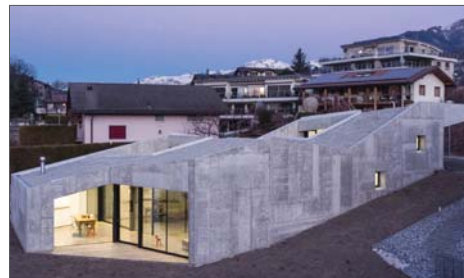
Alps House , Anako Architects Saviese, Switzerland
