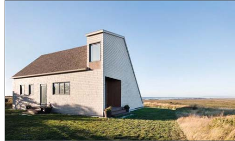
West Dune House , Bourgeois/Lechasseur Architects Quebec, Canada
