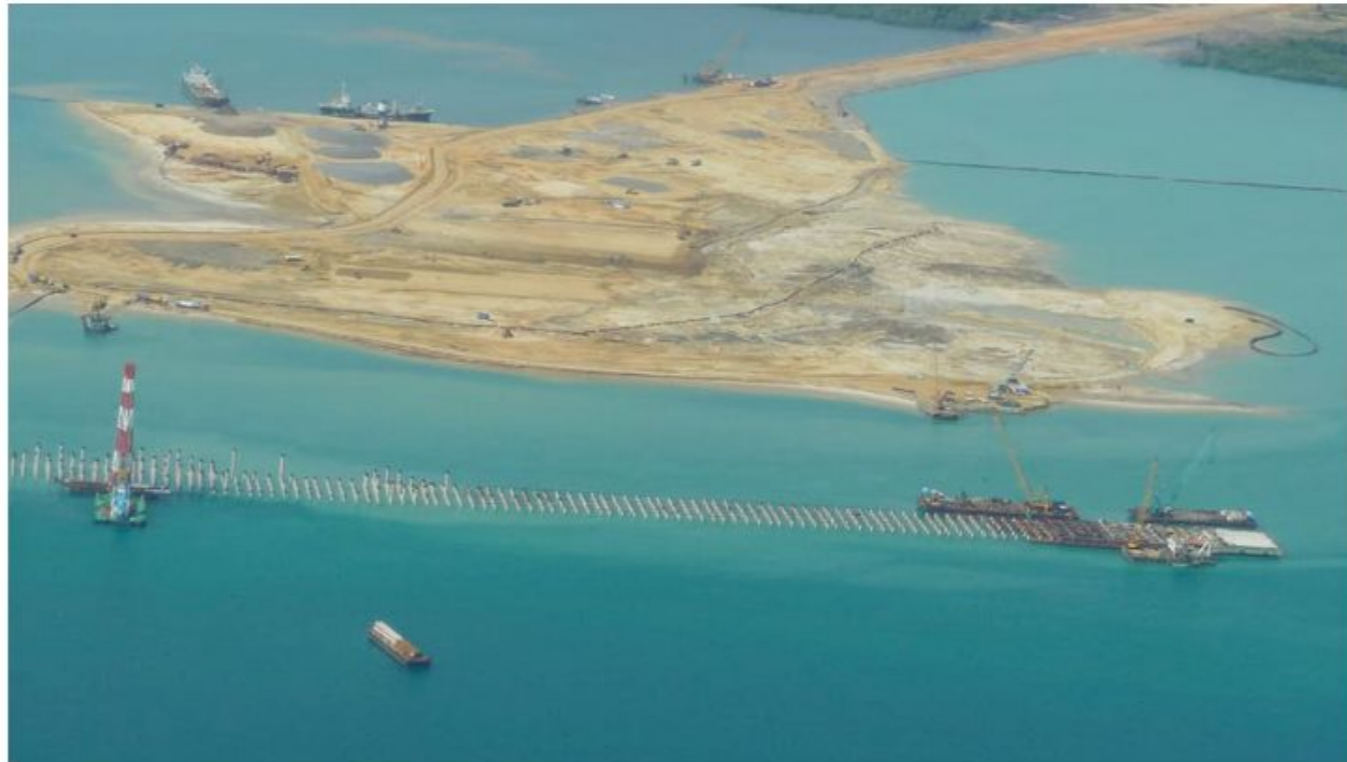
Construction underway of a new port at Lamu, Kenya. Michael Edward Walsh/flickr, CC BY-NC-ND
